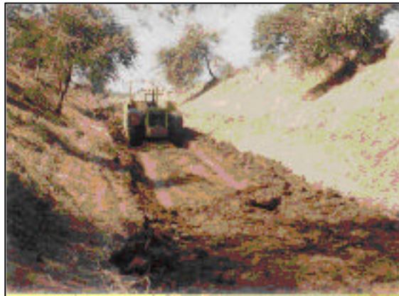
Repairs of Canal in deep cutting portion
