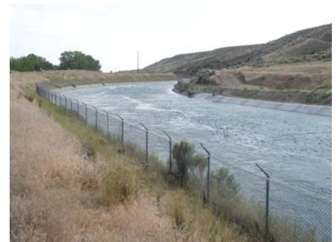
Section of the 50 year-old canal of the Quincy-Columbia Basin Irrigation District, Washington State, USA repaired in 2003 with composite Ethylene-Vinyl Acetate (EVA) liner (0.5 mm) between two non-woven geotextiles. The composite liner was covered with 75 mm poured concrete. Side slopes are 1.5H: 1V. Photos taken of the same section during repair (left) and when the canal back in service (right) [Photo courtesy: Huesker Inc.]
