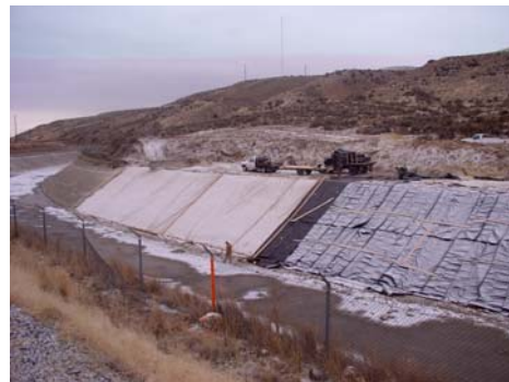
Section of the 50 year-old canal of the Quincy-Columbia Basin Irrigation District, Washington State, USA repaired in 2003 with composite Ethylene-Vinyl Acetate (EVA) liner (0.5 mm) between two non-woven geotextiles. The composite liner was covered with 75 mm poured concrete. Side slopes are 1.5H: 1V. Photos taken of the same section during repair (left) and when the canal back in service (right) [Photo courtesy: Huesker Inc.]
