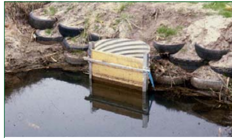
Figure 1. A flash-board riser structure used to implement Controlled Drainage during periods when drainage intensities may be reduced.
