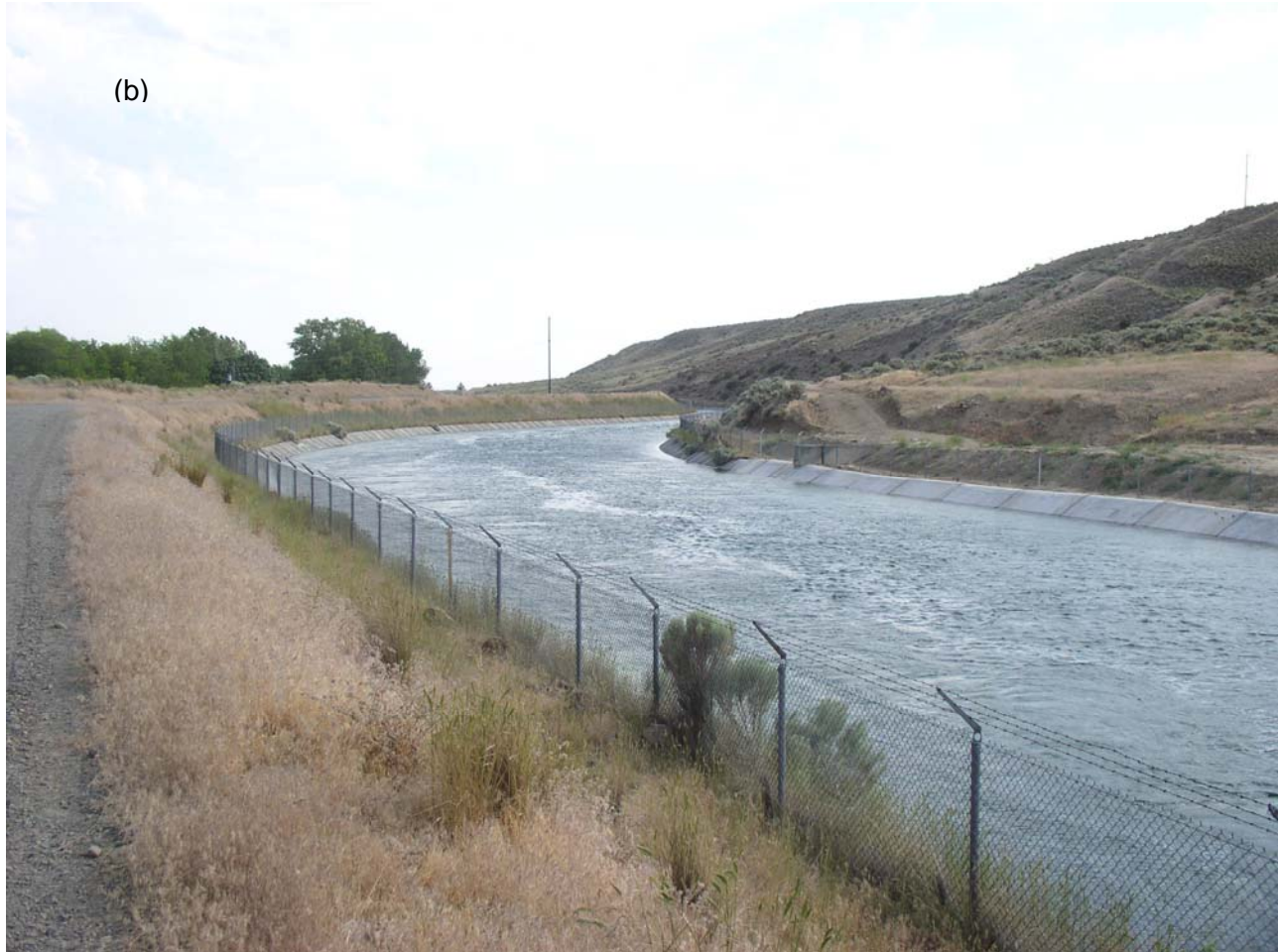
Section of the 50 year-old canal of the Quincy-Columbia Basin Irrigation District, Washington State, USA repaired in 2003 with composite Ethylene-Vinyl Acetate (EVA) liner (0.5 mm) between two non-woven geotextiles. The composite liner was covered with 75 mm poured concrete. Side slopes are 1.5H: 1V. Photos taken of the same section during repair (a) and when the canal back in service (b) [Photo courtesy: Huesker Inc.]
