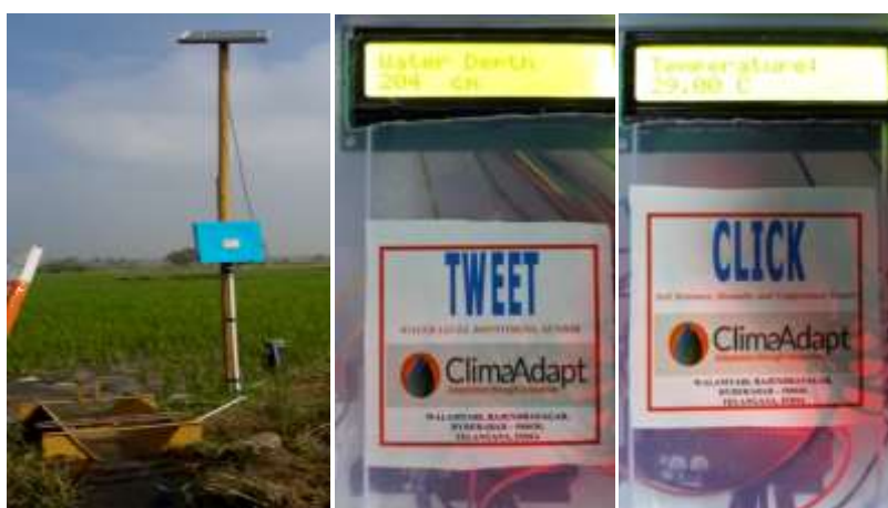
Fig. 2. A tweet sensor installed in the field for measuring water level and flow, soil moisture, temperature and relative humidity with solar power, Kondrapole village, Miryalaguda area, Nalgonda, Telangana
