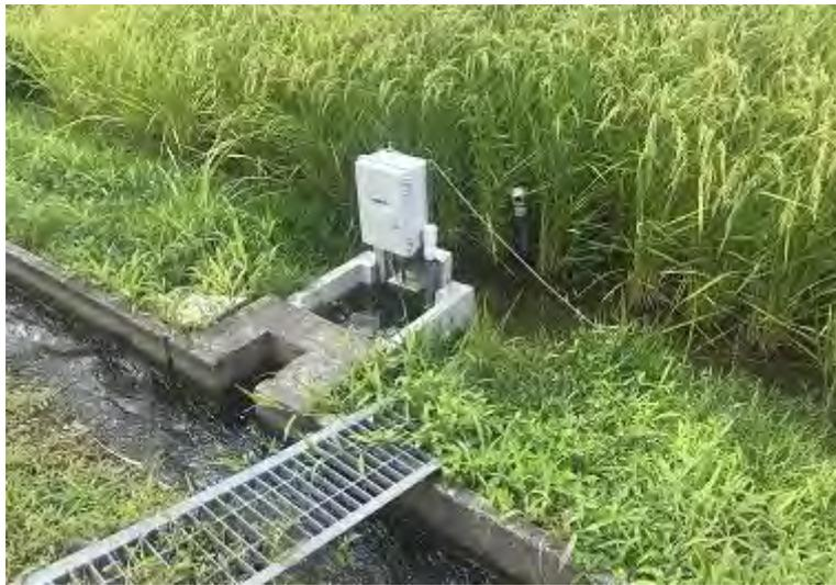
**Figure 1.** Paditch Gate (ICT smart automated sluice gate) installed at plot A.
