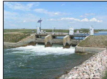
Figure 4. Automated check/drop structure
