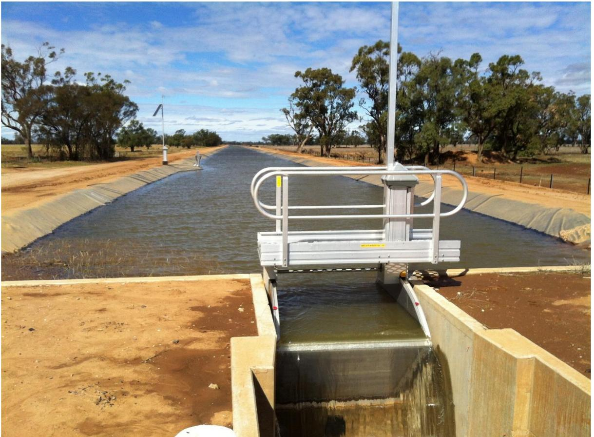
*Photo 1. Lined channel section with Rubicon control gates.*
