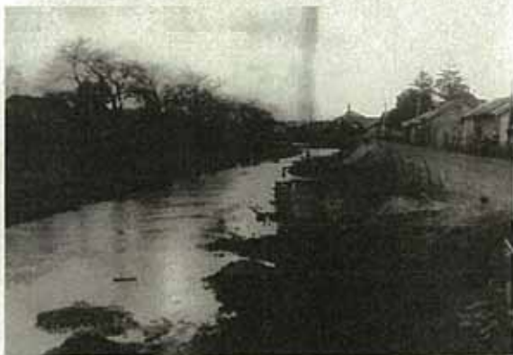
Inaigawa irrigation canal before the implementation of the national project
