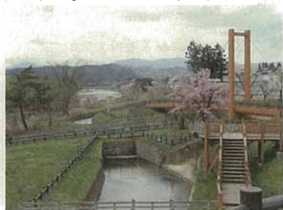
The current Inaigawa irrigation canal (an agricultural park near the entrance of Tengu-yama tunnel, which tells the history of Inaigawa irrigation canal)
