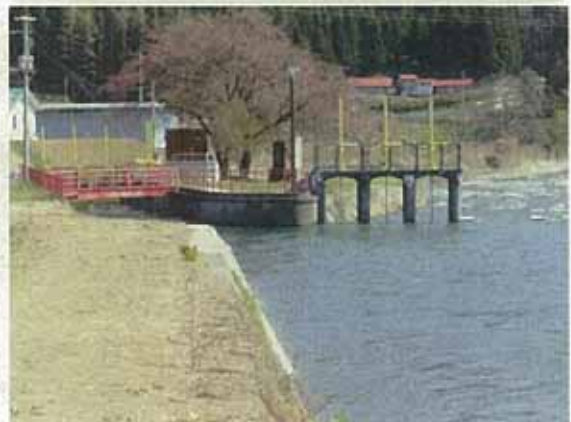
The current Inaigawa irrigation canal (the highest intake in the upriver)
