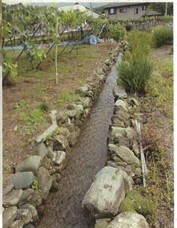
Ogawazeki irrigation canal (branch canal)
