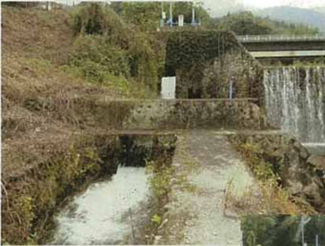
Ogawazeki irrigation canal, water intake (large gate)
