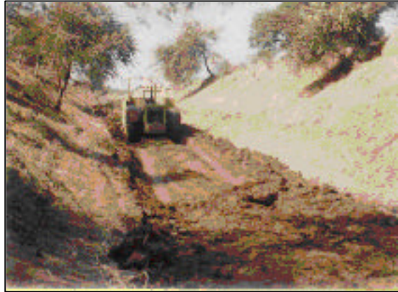
Repairs of Canal in deep cutting portion
