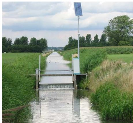
An automated drainage control structure in the central part of the Netherlands
