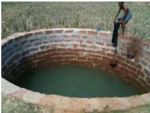
(e) Open well in command area. Farmers pump from these open wells using a small portable pump and lay flat pipe, as shown in (f), OCTMP, Odisha
