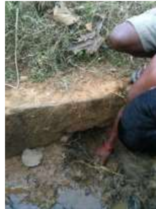
(b) Opening canal outlet by removing the mud
