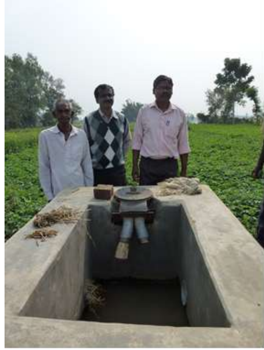
(b) Spout outlet into a chamber, which could be used to measure the flow rate by temporarily closing the outlets and timing how long it takes to fill to a certain (marked) level, Naskarpur Ghantipara Mini RLI scheme, West Bengal
