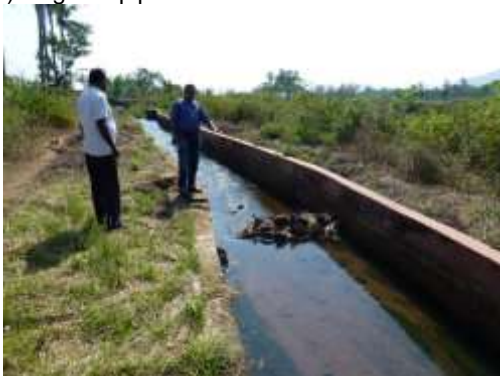
(c) Stones acting as cross regulator in main canal
