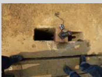
Padlocked sluice gate
