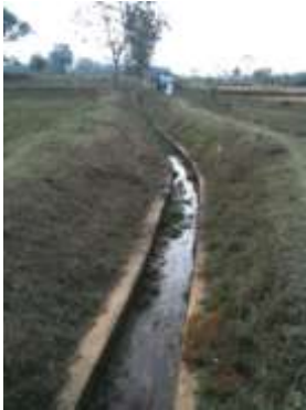
(c) Well-built farmer-constructed canal lining, OCTMP, Odisha.
