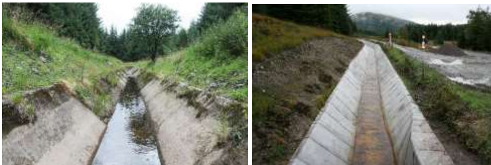
Figure 4. Sections of the Hydropower canal before and after lining with GCCM.
