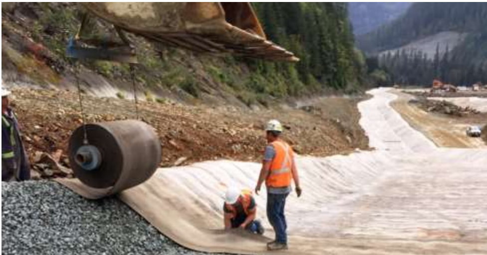
Figure 6. GCCM being installed from a spreader beam at Myra Falls.
