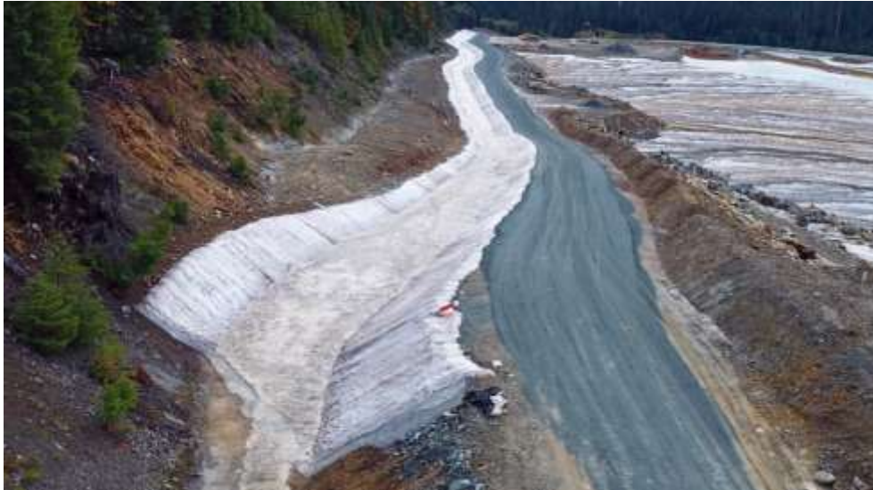
Figure 7. Aerial view of the complete installation with flowing water.
