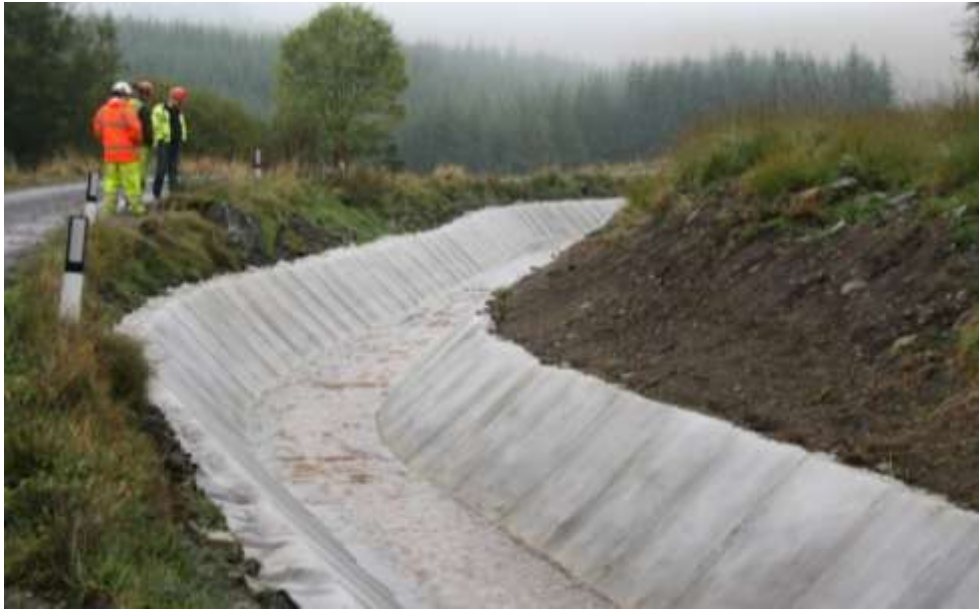
Figure 5. Complete installation showing GCCMs ability to conform to channel curvature.
