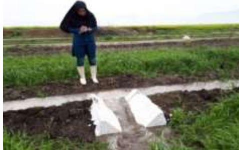
Consumed water rate measurement by using Parshall flume
