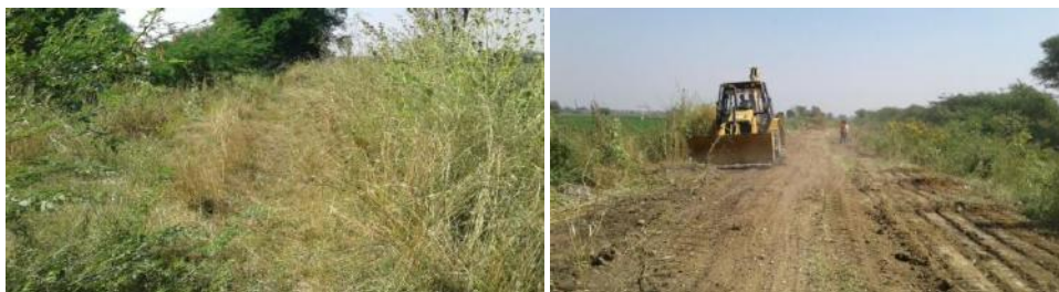
Figure 1. Jungle clearance activities taken up along the length of the Distributory
