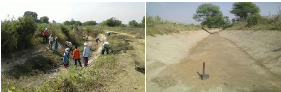
Figure 2. Desiltation works taken up along the Distributory
