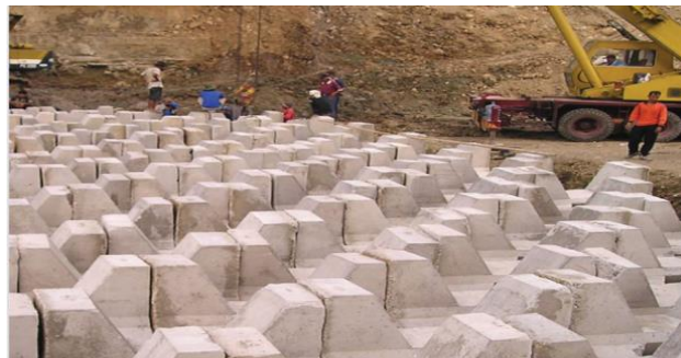
Figure 2. River Bed Protection with Tetrapod in Indonesia (source :Pusair, 2006)
