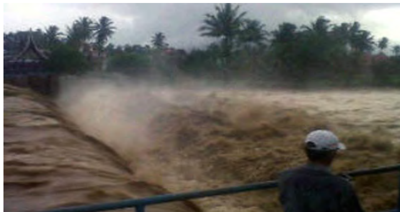
Figure 5. Debris Flood Over The Weir (source :Pusair, 2017)
