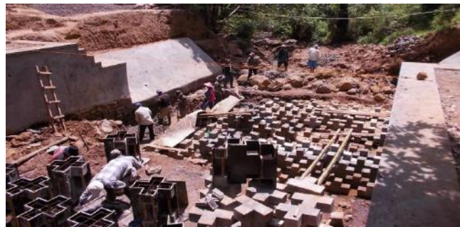
Figure 12. Instalations of the Concrete Modules
