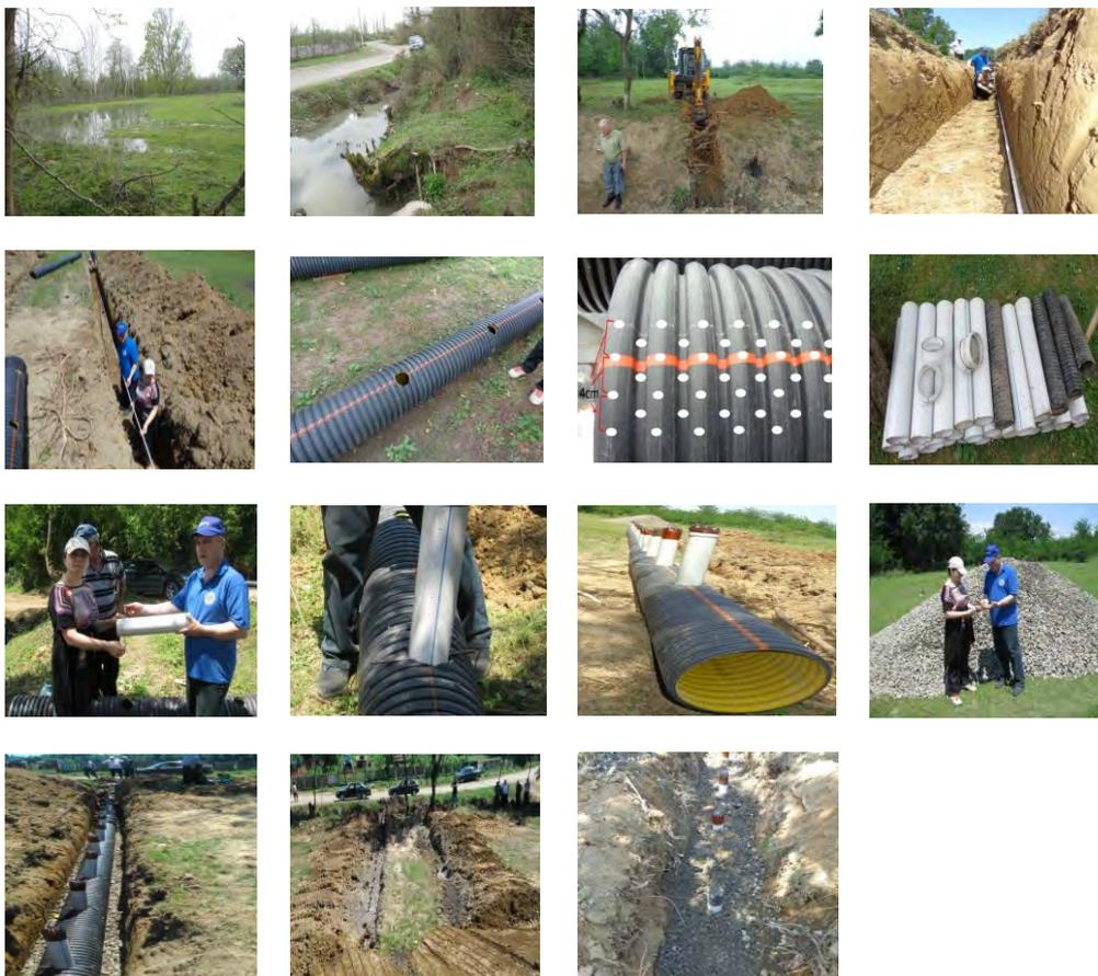
**Figure 7.** Full cycle of the installation of the three-tier drainage.
